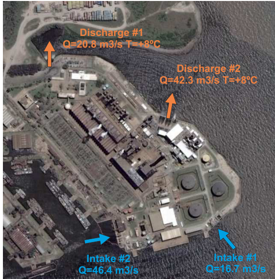
Figure 4. Discharges and intakes at Central Costanera.
